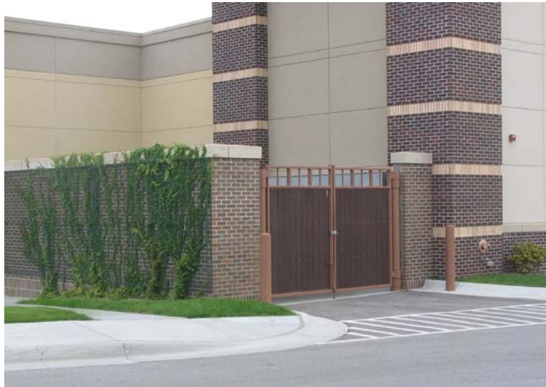
Photo 9—Typical Trash/Service area screen
