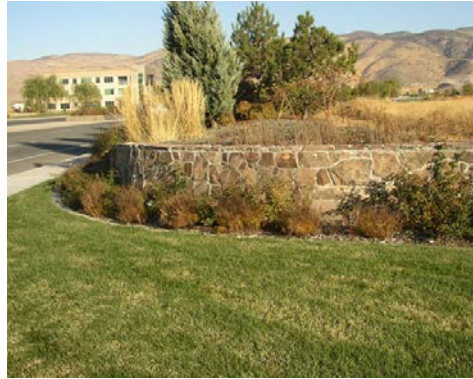
Photo 16—Typical Berm and Lawn Area
